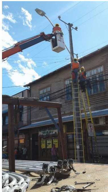
RECAMBIO LUMINARIAS LED
